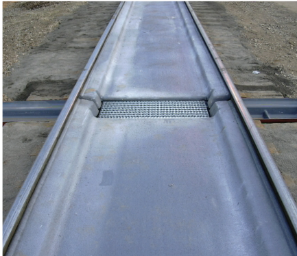
Type III Center Pan Installation
