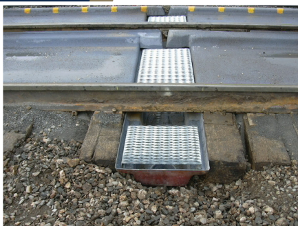
Flat Pan System Install with Crossdrain
