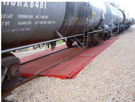
Type III System with Gravel Backfill
