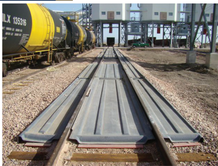
Type V System with Gravel Backfill
