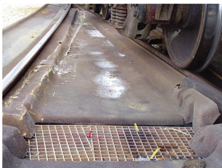
Flat Pan System at Railroad Switch
