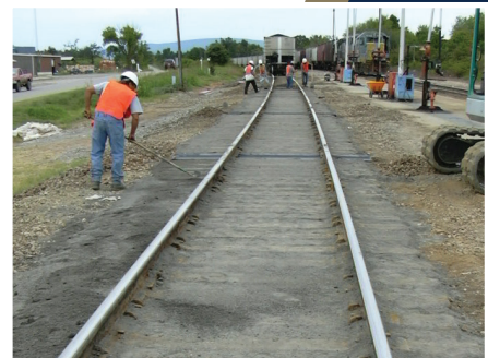
Crossdrain Install and Site Prep
