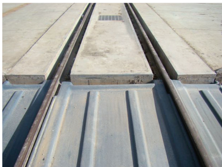
Type V System against Concrete Curb
