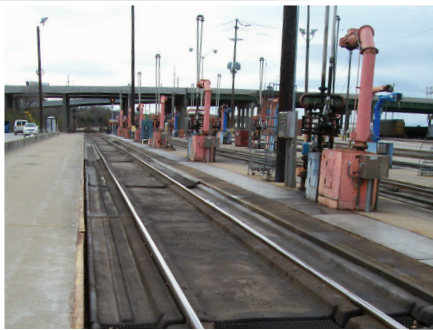
Type IV System with Concrete Curb
